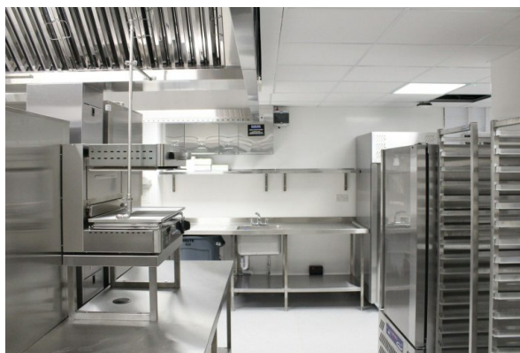
Heating and cooking equipment should be checked against a calibrated reference probe.
